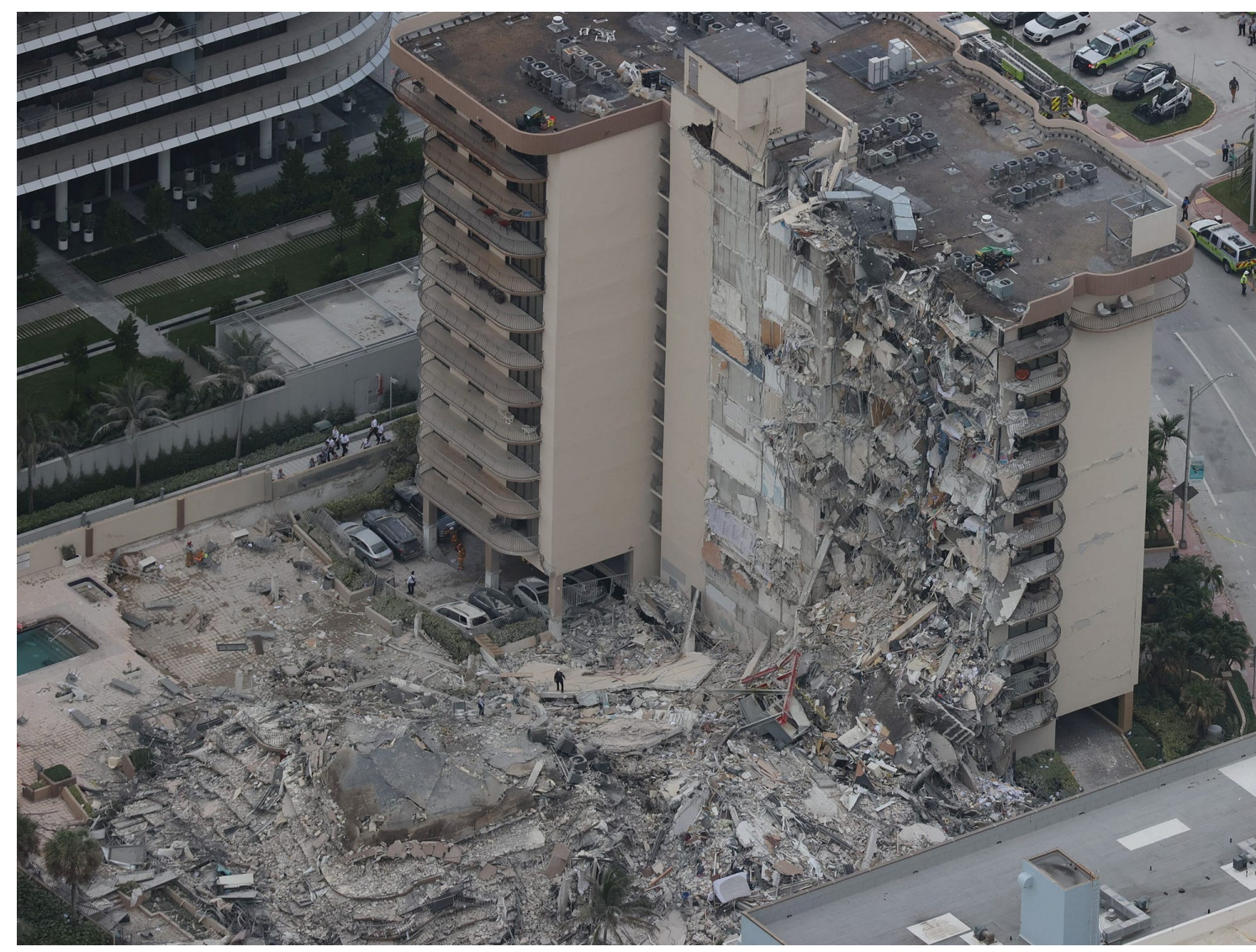
Search and rescue personnel work in the rubble of the 12-story condo tower that crumbled to the ground during a partially collapse of the building on June 24, 2021 in Surfside, Florida. Joe Raedle/Getty Images
